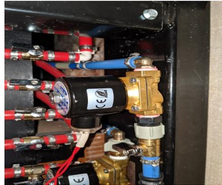
Typical rinse valve and vacuum breaker/check valve installation.
